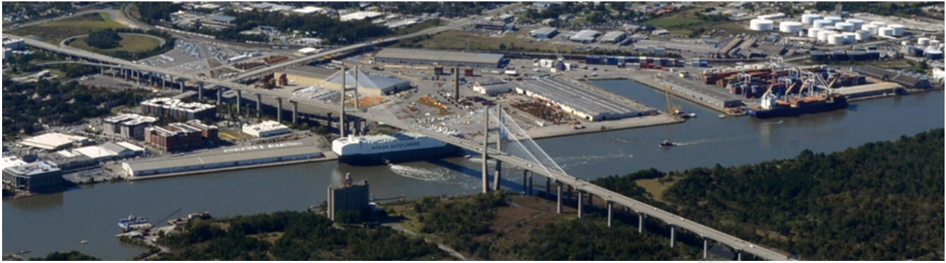
Figure ES-5: Aerial View of Talmadge Memorial Bridge
